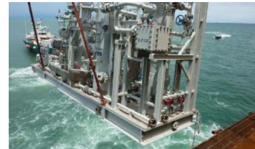
Fuel gas compressor
