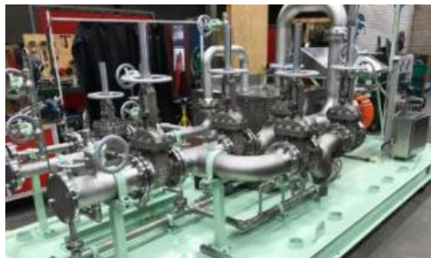
Water injection pump
